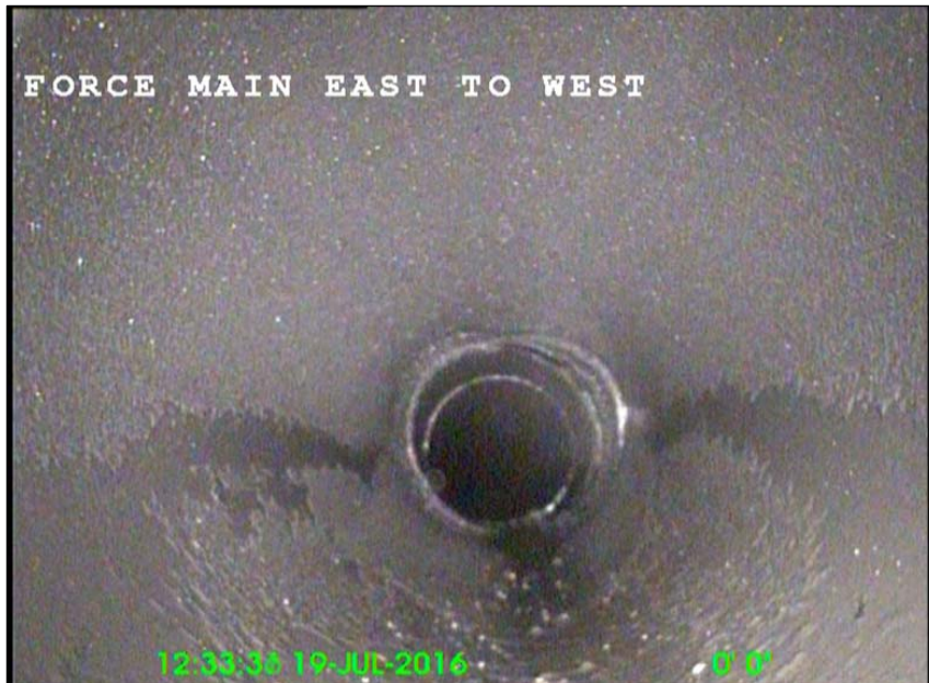
Photo: 1_1_1_A.jpg 0FT, Cleanout Mainline
