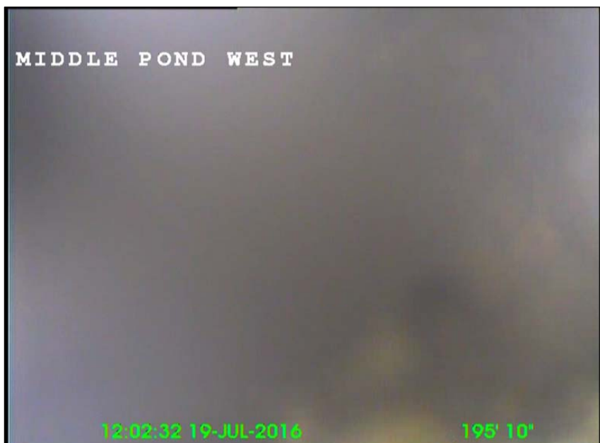
Photo: 4_4_19_A.jpg 195.1FT, General Observation
